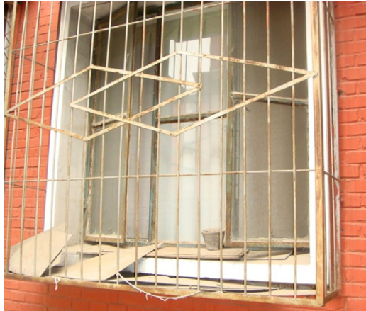
Fig. 5. Window in Ruiguang building in Beijing.
